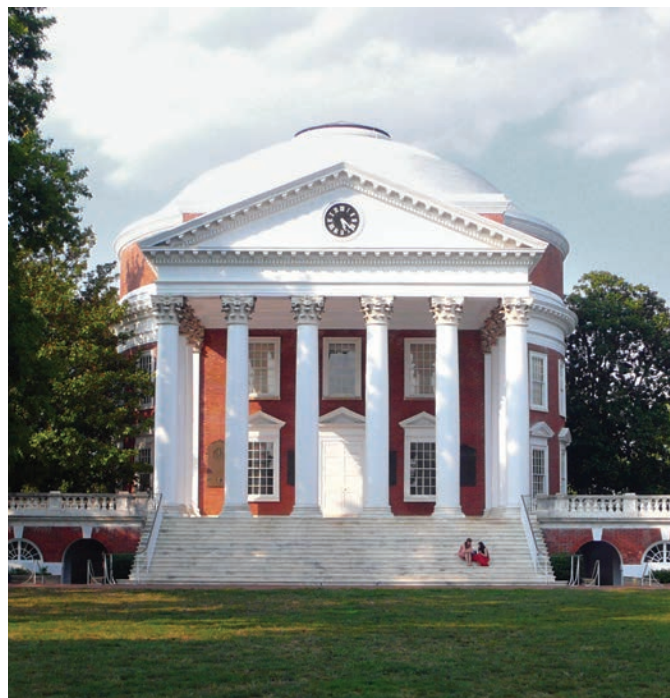
The Rotunda was the site of UVA's first library and remains a central point on grounds. Source: UVA
