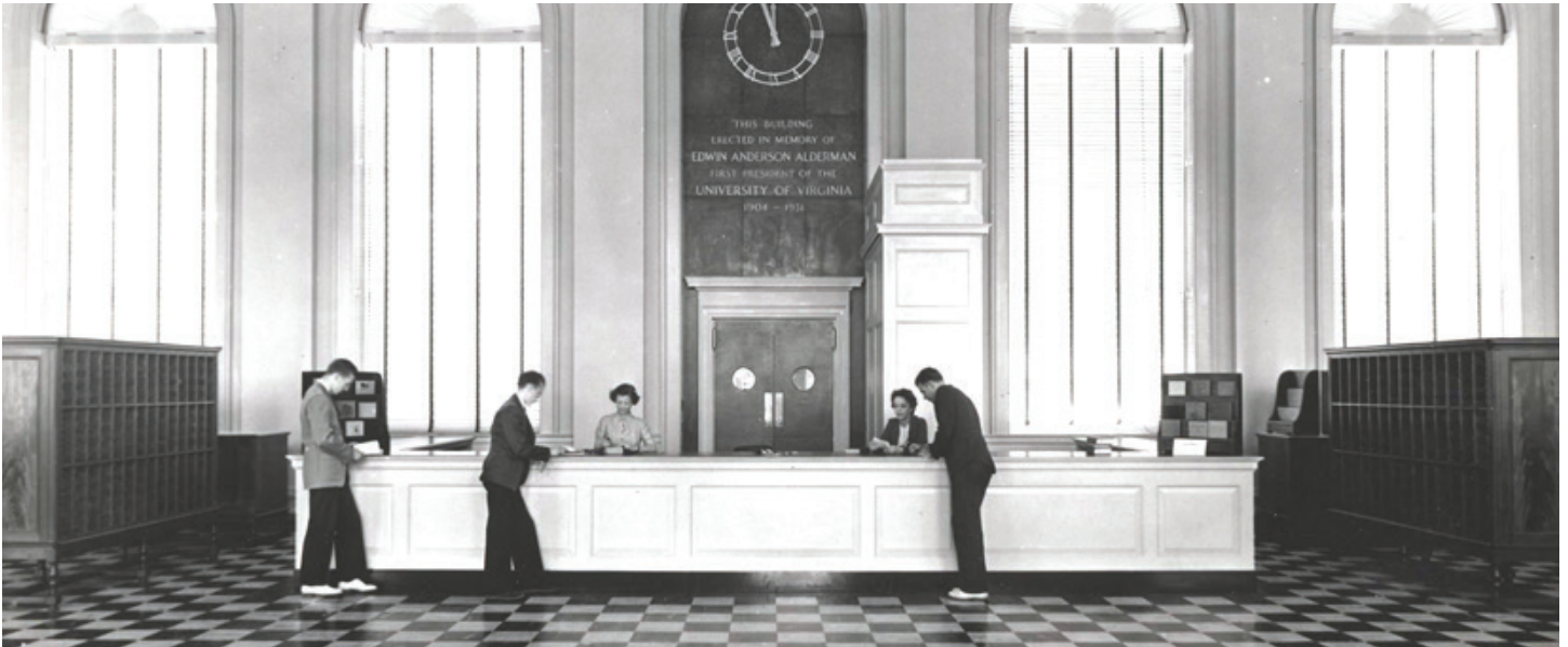
Alderman Library in 1938, showing controlled access to stacks
